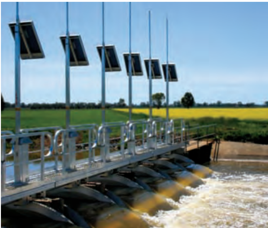
Solar powered equipment and accompanying software are used to regulate the flow of water through the open channels.
